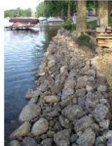
Here is a picture of a typical lake shore rip rapping with native plantings project on a local lake. Morgan Lloyd
